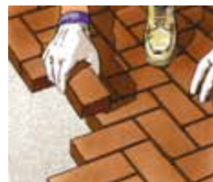
5. Lay Paving Stones
